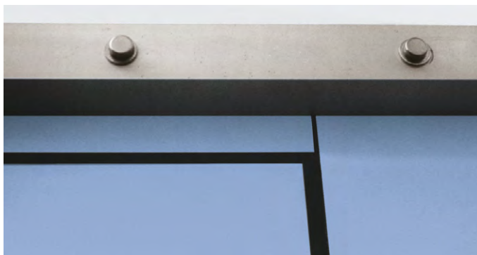
SUPPORT AREA FOR INWARDS OPENING DOORS A MINIMUM OF 80 MM HIGH, IN ORDER TO BE ABLE TO HANG THE DOOR, DIMENSION A.
